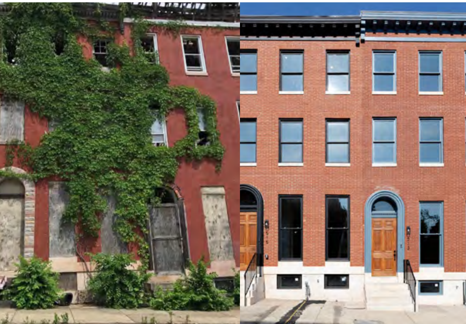
Side by side, the homes reinvested by Parity are transformed for historically redlined communities. PHOTO CREDIT: Bree Jones
